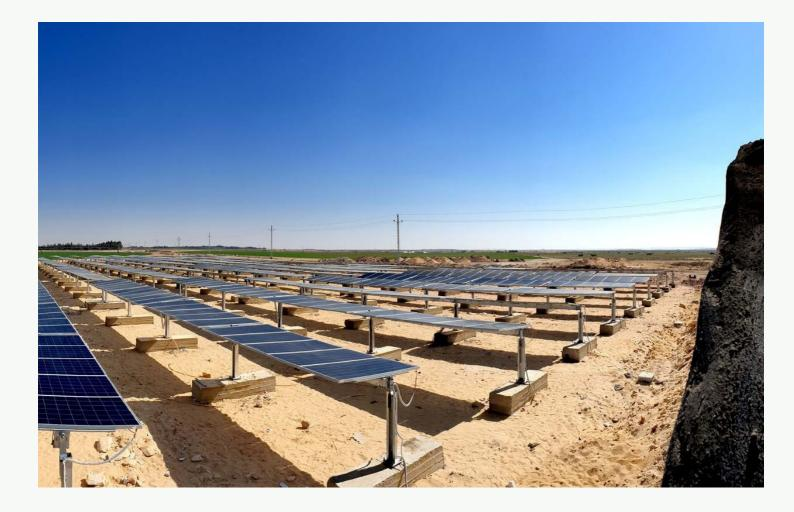
Groups of solar panels are located next to each field. It takes 21 solar panels per field to pump the water and operate the pivot.
