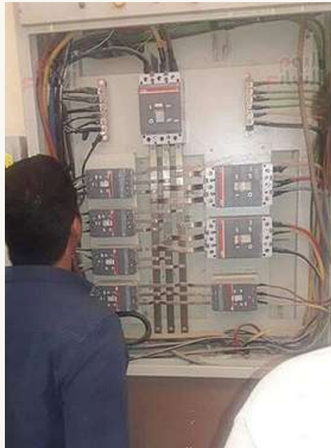
Visitors inspecting the school's electrical box.
